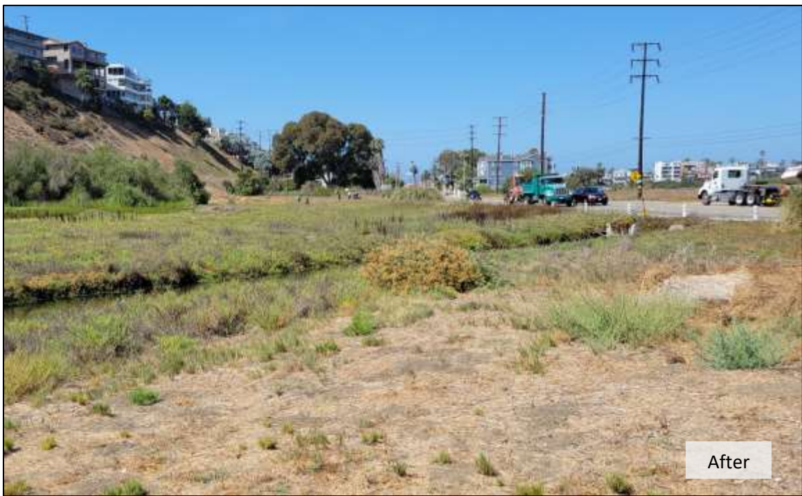
Figure B9. Site photograph prior to restoration (left, September 2016) and after restoration activities (right, July 2021).
