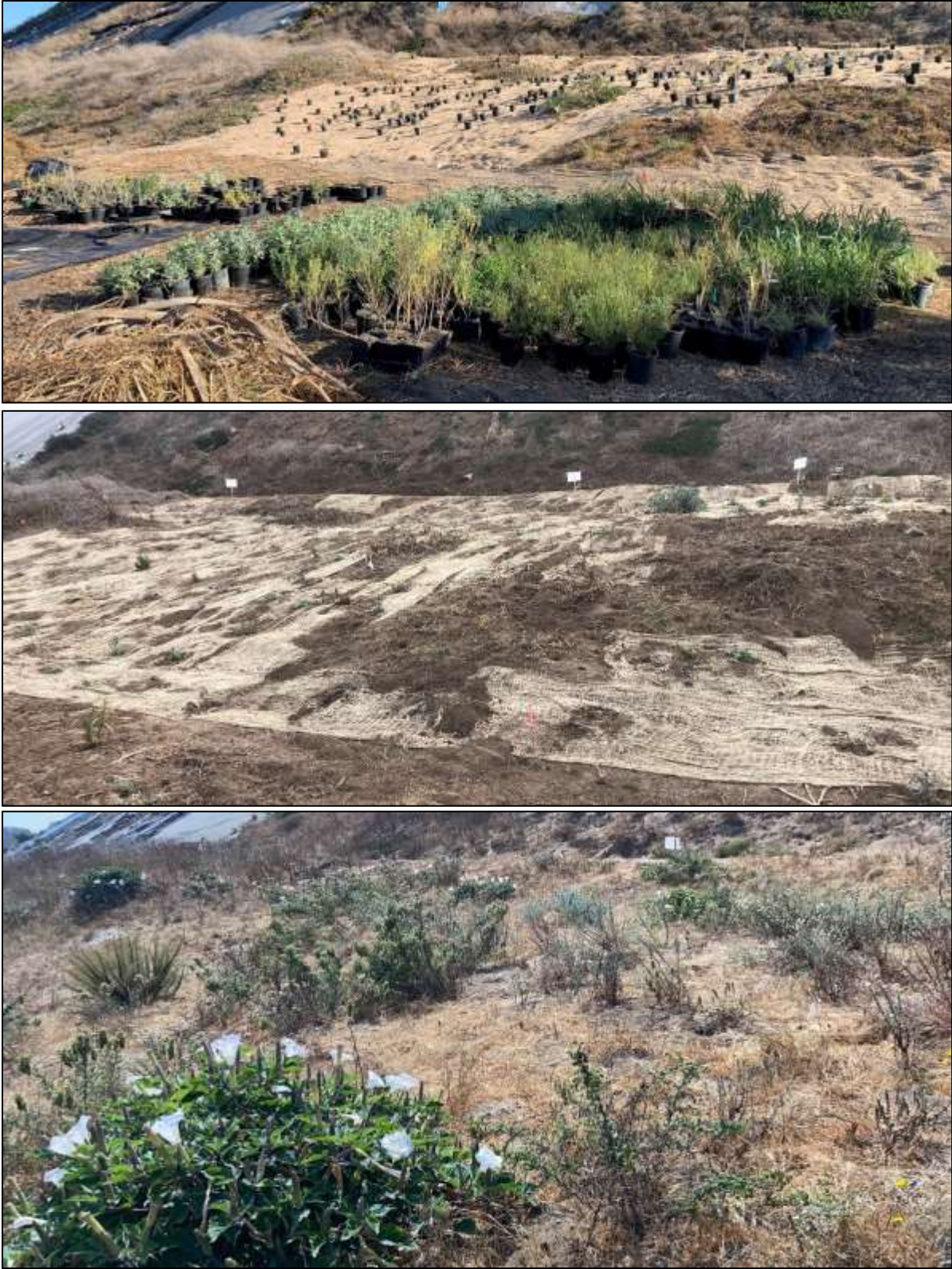
Figure 4. Photographs of hillside restoration activities planting native container stock vegetation (top, 18 November 2020), approximately one month after planting (middle, 23 December 2020), and approximately seven months after implementation (bottom, 7 July 2021).
