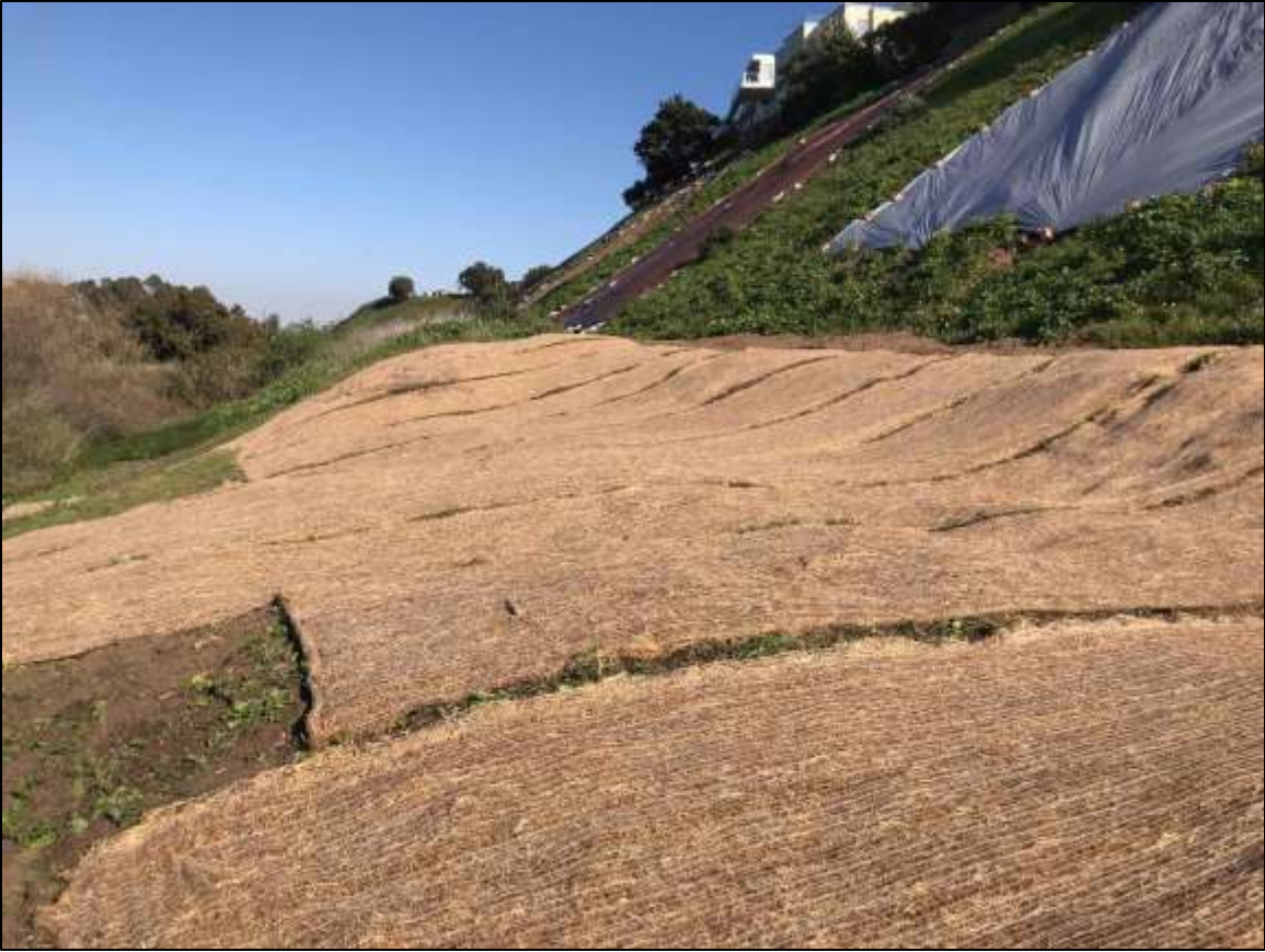
Figure 9. Photograph of installed erosion control matting completed on 8 February 2019.
