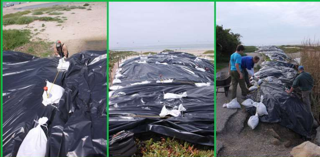
Left: staff suspends sandbags from stakes and lines to hold the plastic sheeting in place on a steep slope. Middle and right: finished sections.
