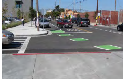
Dashed green lane striping crossing from on-street bicycle boulevard to multi-use path along the 9 th Street Bicycle Boulevard in Berkeley, CA.
