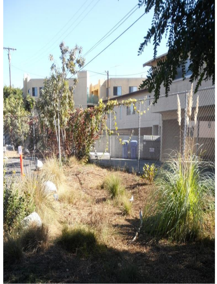
Detention basin with native drought tolerant plants capture rain water and allows the rain water to seep into the ground.
